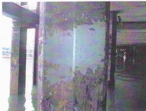
Plate 1. Area of pile cleaned for inspection
